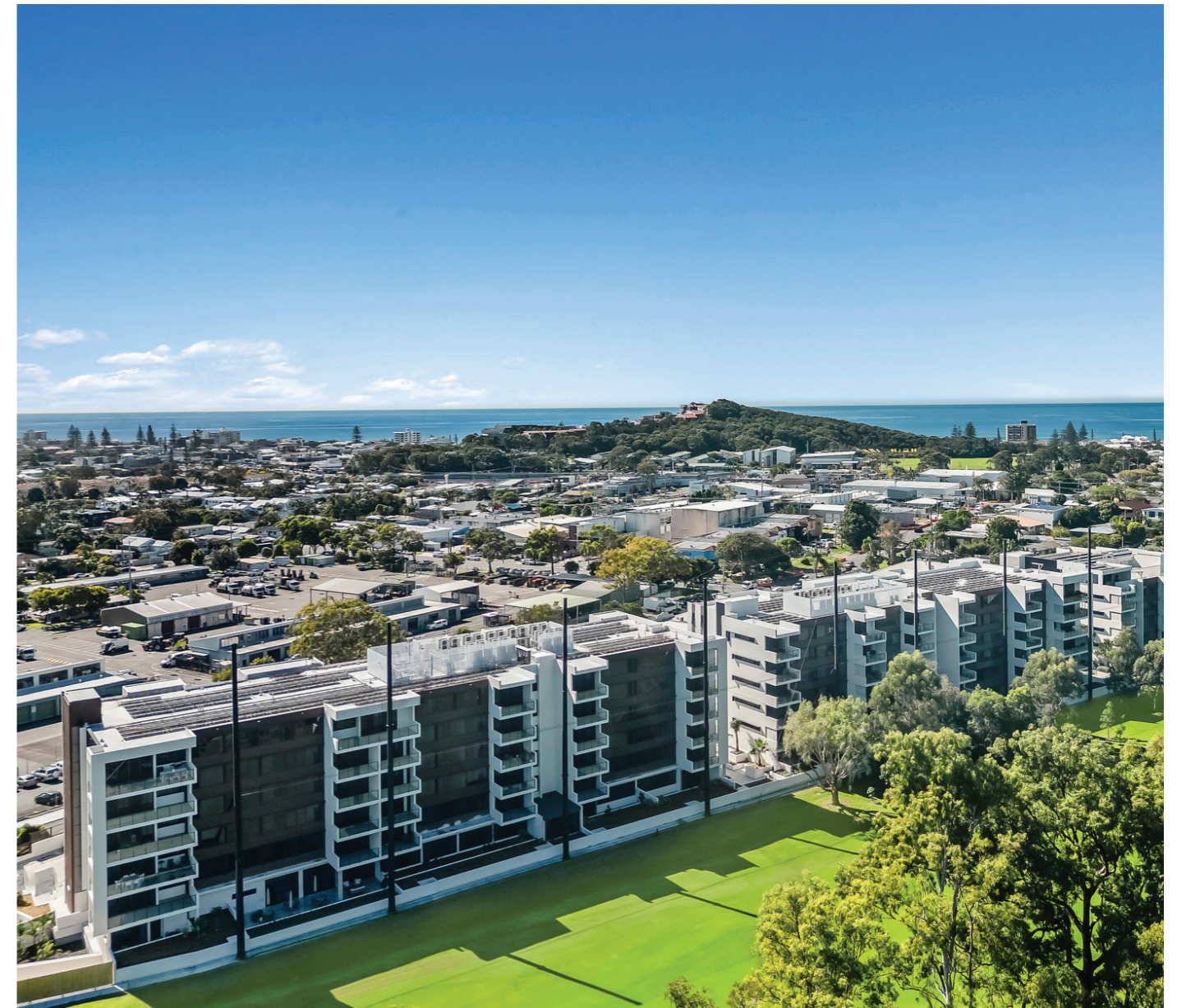
Built along the 10th Fairway of Burleigh Golf Course, The Verge offers residents unparalleled views and connection to nature.
